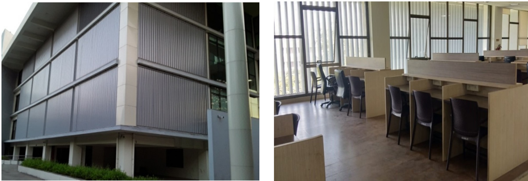
Fig. 4: Louvers to Manage Sunlight
